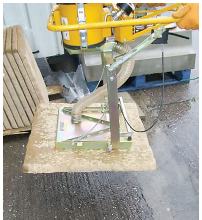
Figures 17 and 18. Vertically stacked paving slabs on a shipping pallet can be lifted, turned to a horizontal position and placed with a vacuum device.
