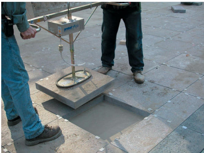
Figure 14. Two-person vacuum lift for paving slabs
