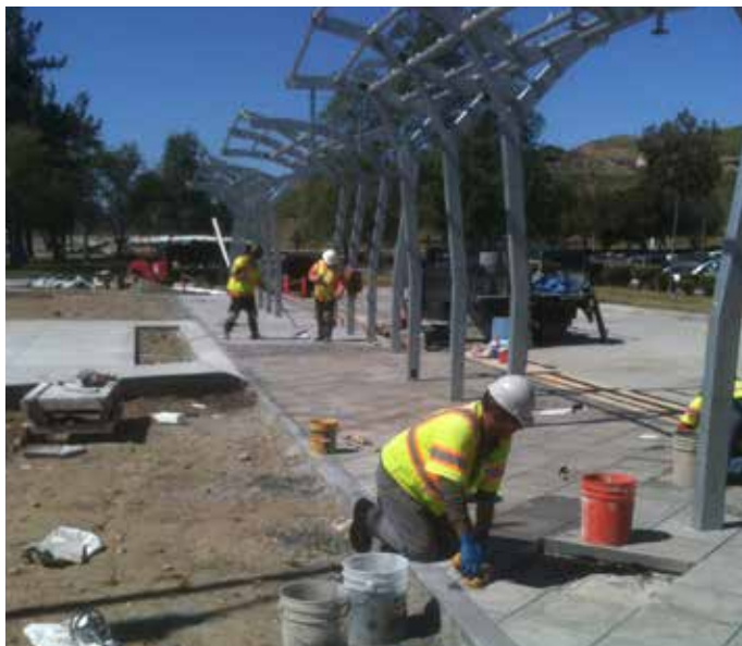
VP Joint Grout - Premium (E Street Project)
