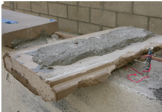
The added flexural bond was stronger than the precast concrete itself. Conventional polymer cement mortars had failed in bonding these cantilevered wall caps.
