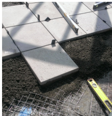
DECK MUD - POLY WITH VBM BONDER SLURRY COAT. GROUTED WITH VP JOINT GROUT PREMIUM
