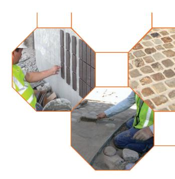
Poly Deck Mud and Deck Mud are dry, factory blended mortars designed to produce high strength thick mortar beds. OBP Poly Deck Mud has added polymers providing additional strength, water repellant properties and efflorescence protection for the most demanding applications. The water repellant properties can reduce or eliminate moisture migrating to the paver from the sub base. They are a blend of Portland Cement, washed masonry sand and proprietary admixtures.
