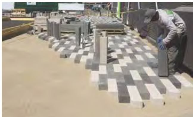
Figure 6. Installing planks on uncompacted bedding sand.
