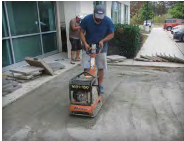
Figure 5. Precompacting the bedding sand
