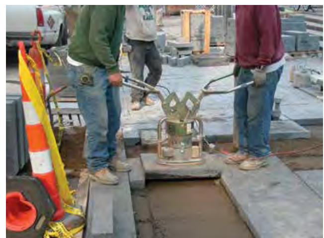
Figure 15. Two-person vacuum lift for larger paving slabs.
