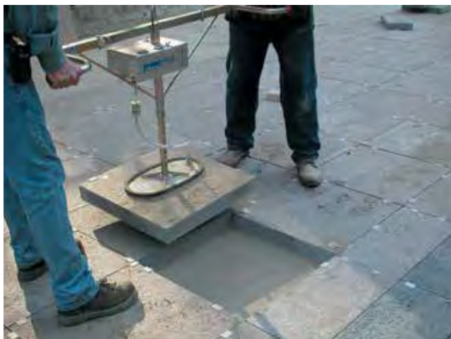
Figure 14. Two-person vacuum lift for paving slabs
