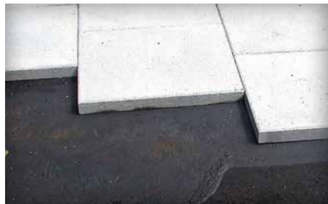
Figure 8. Sidewalk application illustrating the neoprene adhesive on an asphalt bedding layer under paving slabs
