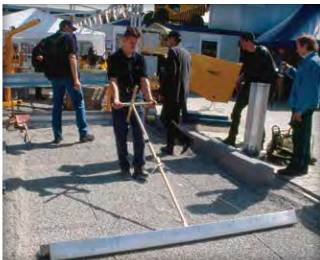
Figure 24. Manually screeding the No. 8 stone setting bed.
