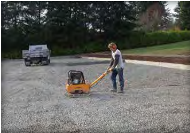
Figure 21. A 13,500 (60 kN) vibratory plate compactor is used on this ASTM No. 57 stone base.
