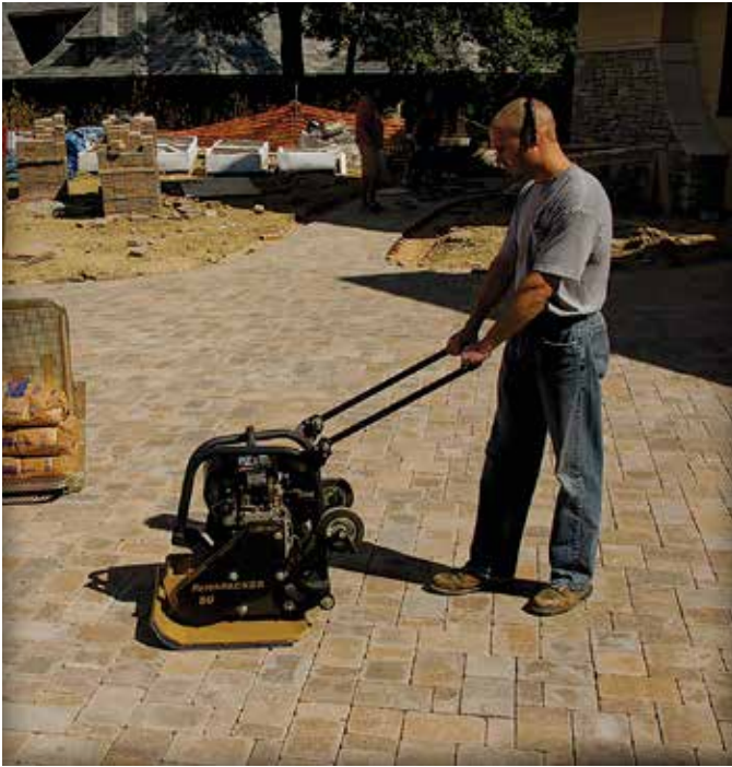
Figure 9. Compacting the pavers and bedding sand.
