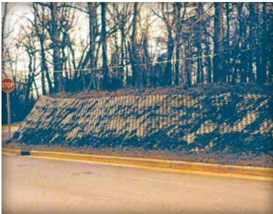
Figure 9. Embankment stabilization
