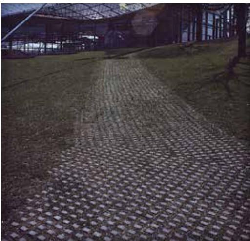
Figure 6. Service access lane
