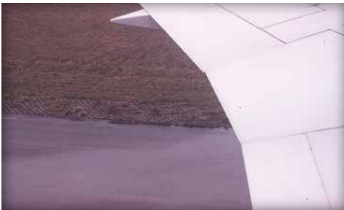
Figure 11. Airfield taxiway shoulder
