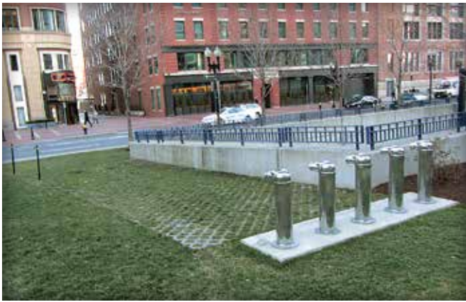
Figure 7. Emergency access lane for fire trucks
