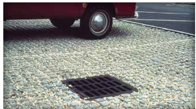
Figure 16. Concrete grids with aggregate in the openings
