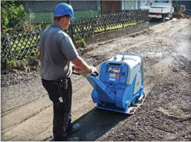
Figure 4. Base compaction with a reversible plate compactor.
