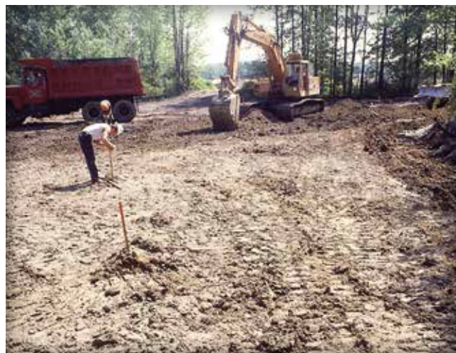
Figure 1. Excavation of the soil subgrade and placing grade stakes.
