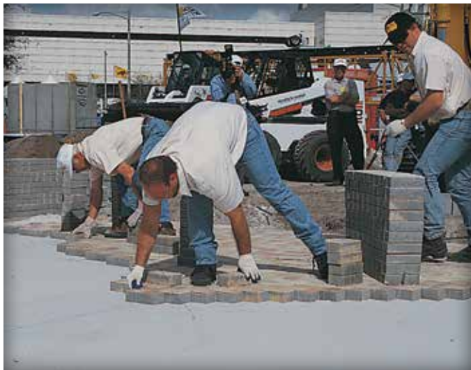
Figure 7. Placing the concrete pavers.
