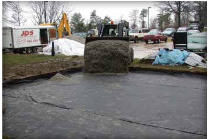
Figure 3. Application of the geotextile under aggregate base.
