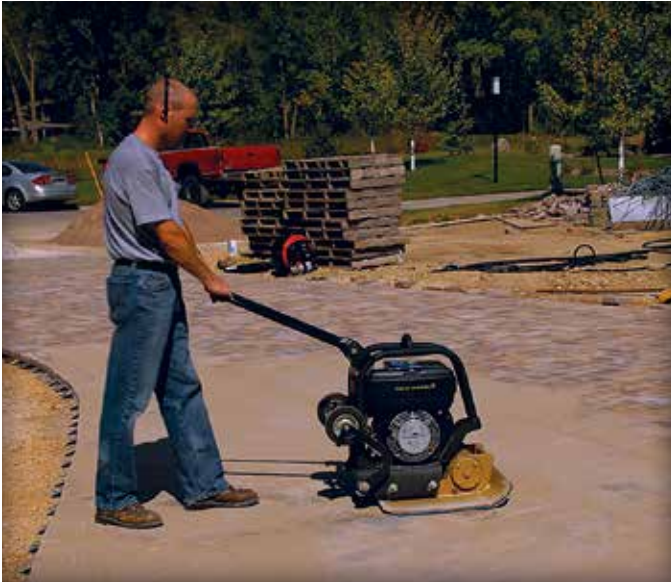
Figure 11. Vibrating sand into the joints.
