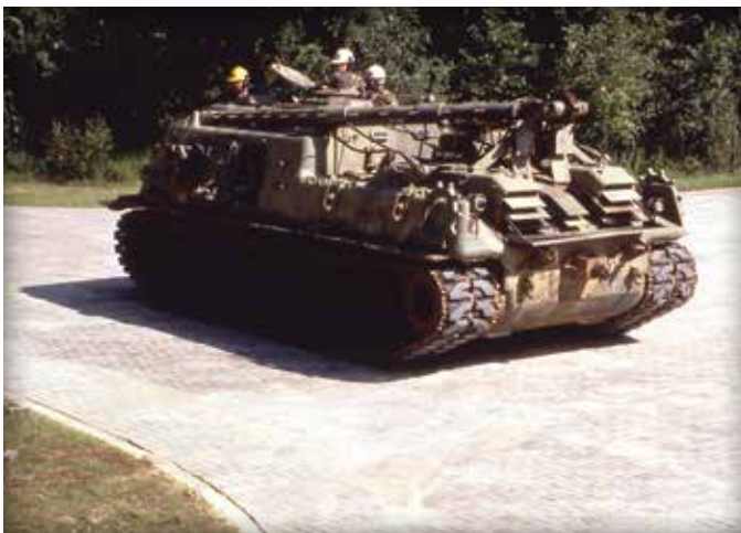
Figure 13. The completed paved area from Figure 12 receives tank traffic at the U.S. Army Proving Grounds in Aberdeen, Maryland.
