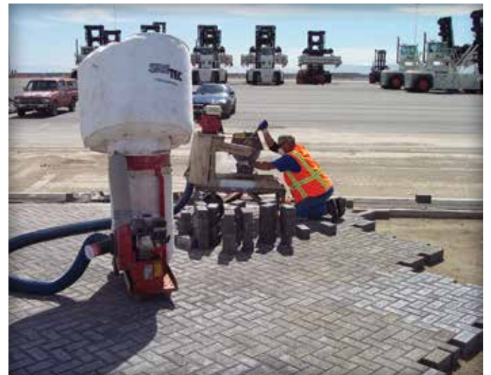
Figure 8. Saw cutting pavers.
