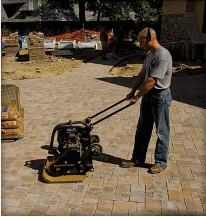
Figure 9. Compacting the pavers and bedding sand.
