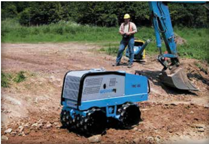
Figure 2. Compacting the soil subgrade.
