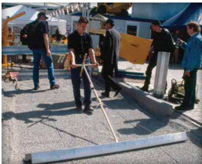
Figure 24. Manually screeding the No. 8 stone setting bed.
