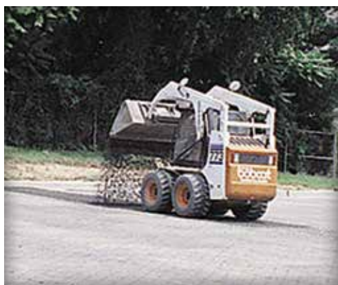
Figure 28. Various methods of filling and sweeping PICP joints.
