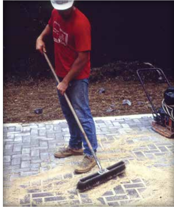
Figure 10. Spreading and sweeping joint sand.
