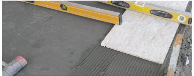
MINUTES. USE THE CORRECT SIZE NOTCHED TROWEL TO MAKE SURE VENEERS ARE FULLY EMBEDDED (100% COVERAGE). PLACE TILE OR VENEERS INTO THE WET MORTAR AND BEAT INTO PLACE. DO NOT APPLY TO SKIMMED OVER MORTAR. BACK BUTTER LARGE VENEERS. ASSURE FULL COVERAGE AND BOND BY PERIODICALLY REMOVING AND INSPECTING THE BACK OF TILE. TILE OR VENEER THAT HAVE BEEN SET FOR MORE THAN 10-15 MINUTES CANNOT BE RE-ADJUSTED.
