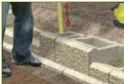
At each 8 in. (200 mm) lift, compact the block cores with the end of a shovel, and the area directly behind the block with a plate compactor per the procedures described in this guide.
