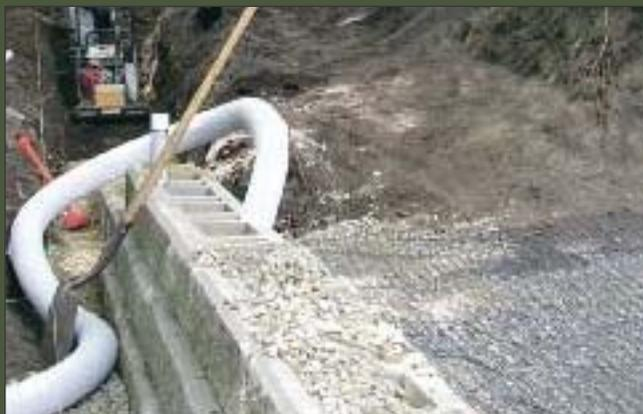
Use a drain pipe to route water from behind the wall. Attach tee fittings at 30 ft. to 50 ft. (9 to 15 m) intervals and direct the drains out through the wall face.
