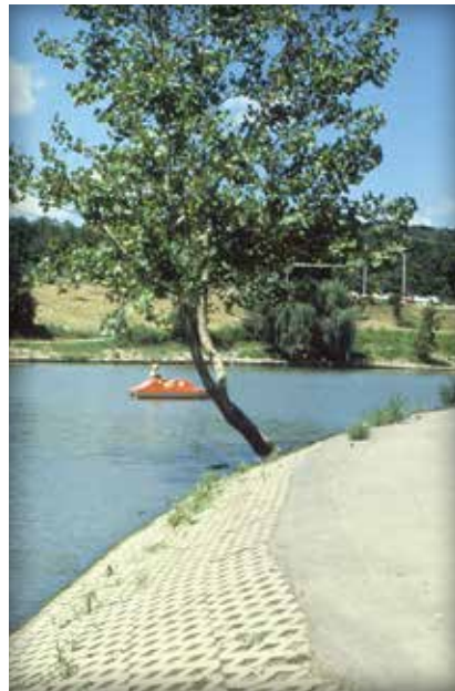
Figure 4. Lakeside stabilization
