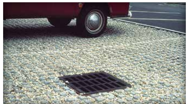
Figure 16. Concrete grids with aggregate in the openings
