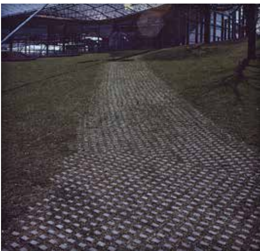
Figure 6. Service access lane
