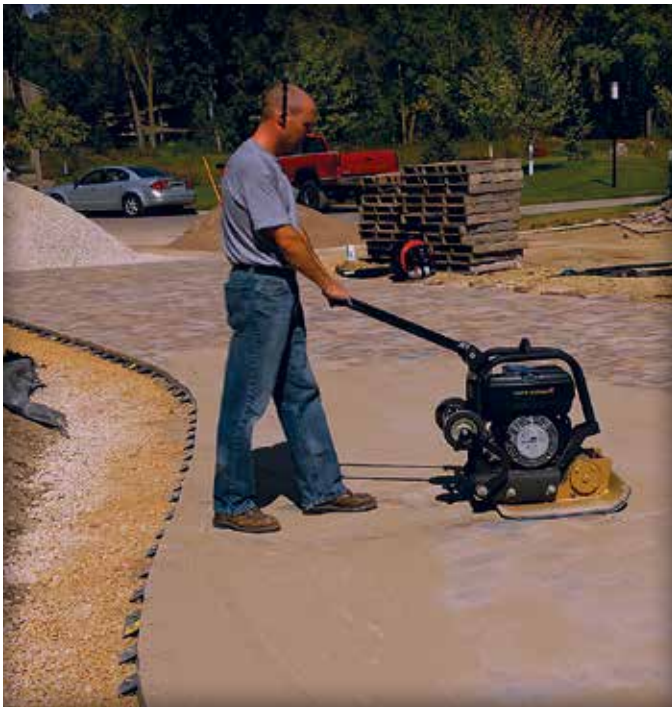
Figure 11. Vibrating sand into the joints.
